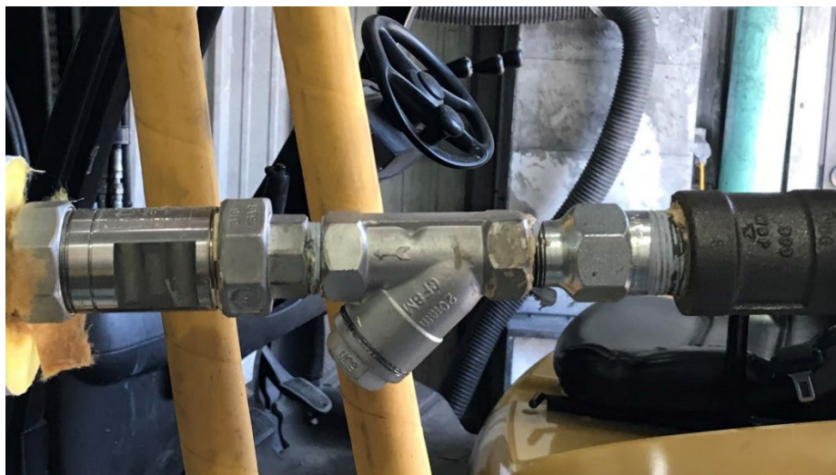
Figure 3. Venturi Steam Trap Installed
