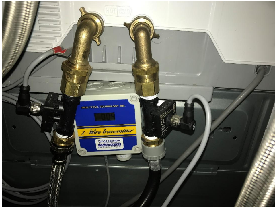
Figure 9: Peoples RO-3 Temp and Flow Meters and Ambient Ozone
