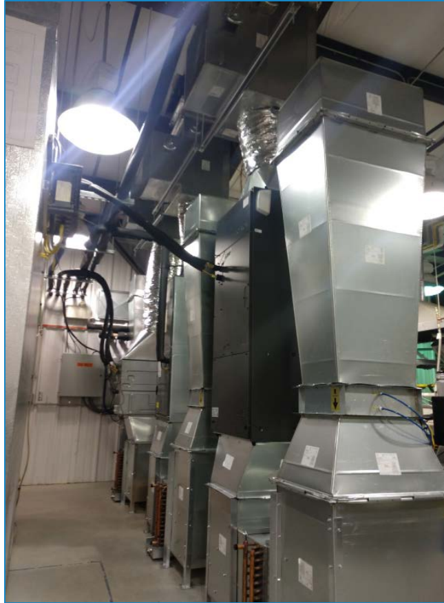
Figure 17 – Space Heating and Cooling Simulator Infrastructure in the VTH Laboratory
