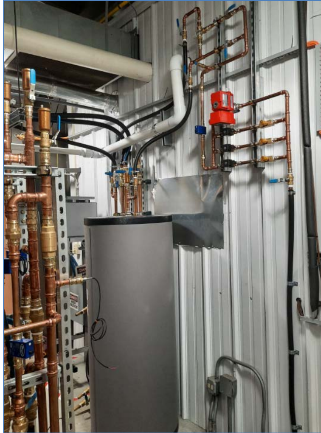
Figure 21 – Water Heating Simulator Infrastructure in the VTH Laboratory
